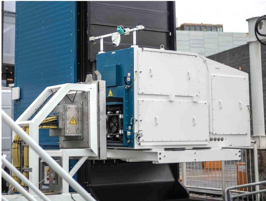
Figure 64: Cavotec 2 x 1,900 kW, 1000VDC SBC system for e-ferry in Nesodden, Norway, with 690VAC vessel charging (source: Cavotec)
