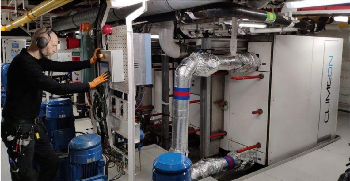
Figure 76: Climeon HeatPower system, installed on Viking Line's *Glory*, IMO no. 9827877 (source: gcaptain.com [C19])
